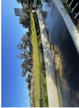
Concrete swale
