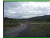
Monitoring, Maintenance and Fire Control Access around the site
