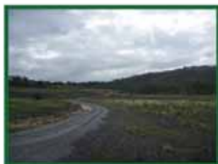
Monitoring, Maintenance and Fire Control Access around the site
