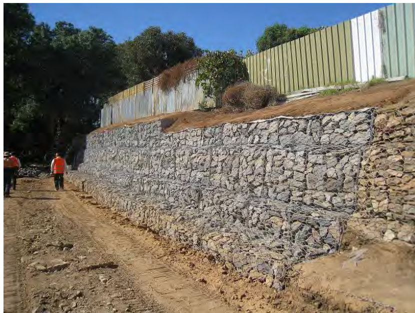
Gabion retaining wall constructed by West Torrens Council in 2012
