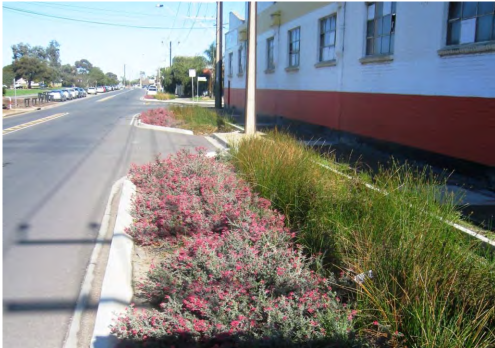
Typical rain garden (WSUD application) in West Torrens Council area
