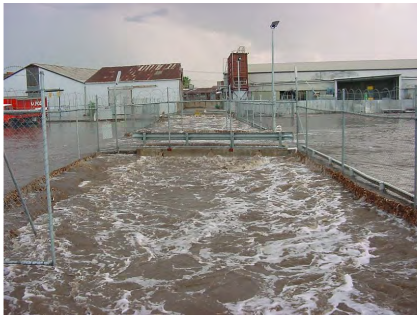
Keswick Creek in Mile End with high stormwater flow and localised flooding
