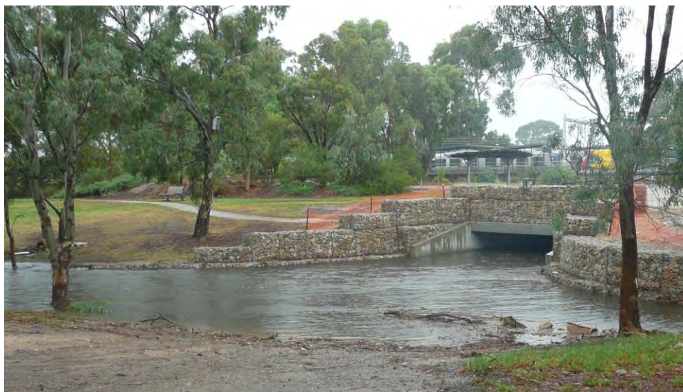
DPTI culvert outlet into Brown Hill Creek in Forestville Reserve (February 2014)
